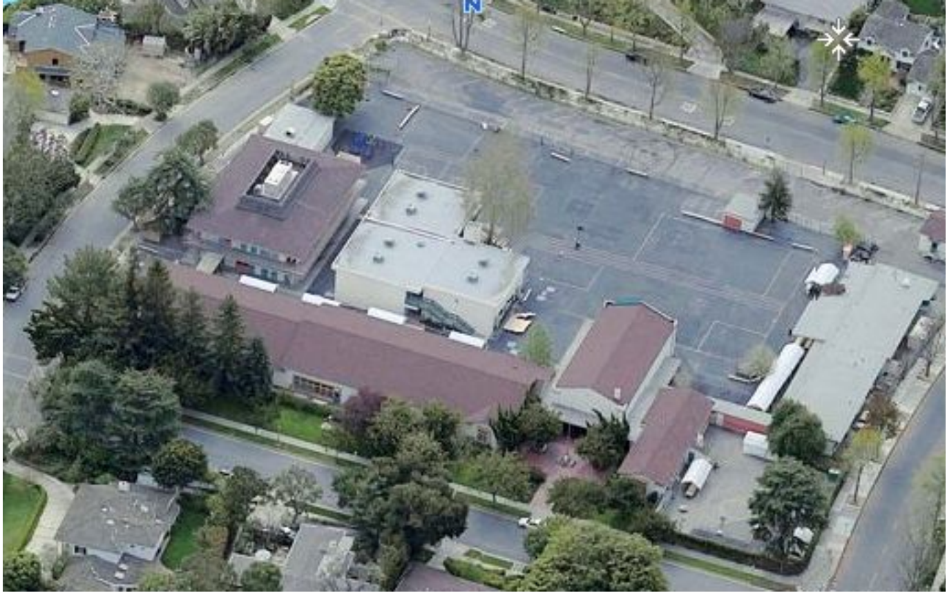
Aerial shot looking South. Also 2005?
