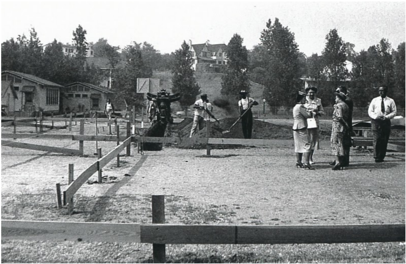
Another view of the construction.
